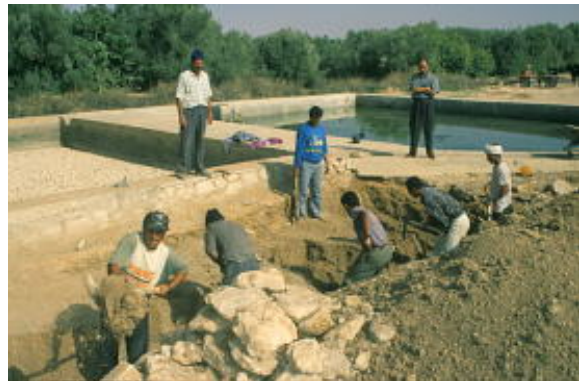
Many Water Harvesting structures are being rehabilitated in Morocco
